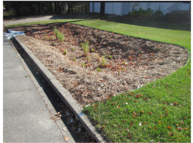
Example of compost-enriched engineered media in a bioretention practice. Image from MPCA's Flickr website. (https://www.flickr.com/photos/mpcaphotos/albums/72157660843839122)
