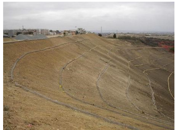
Fiber rolls along slope. Source: Tetra Tech.
