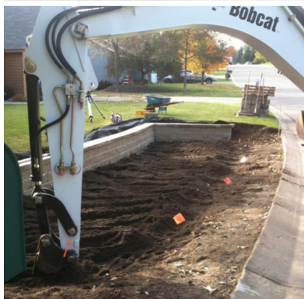
Example of subsoiling and incorporation of compost and sand. Note the equipment is kept out of the practice.
