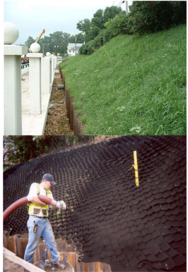
Application of compost blanket roadside County Road 41 in Carver County. Top image - before and during application. Bottom image - after application of compost blanket.
