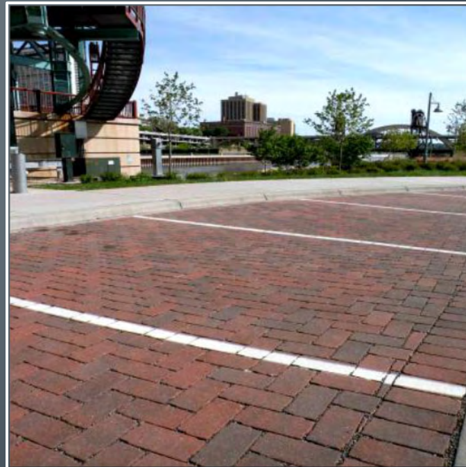
Permeable interlocking concrete pavement (PICP)
