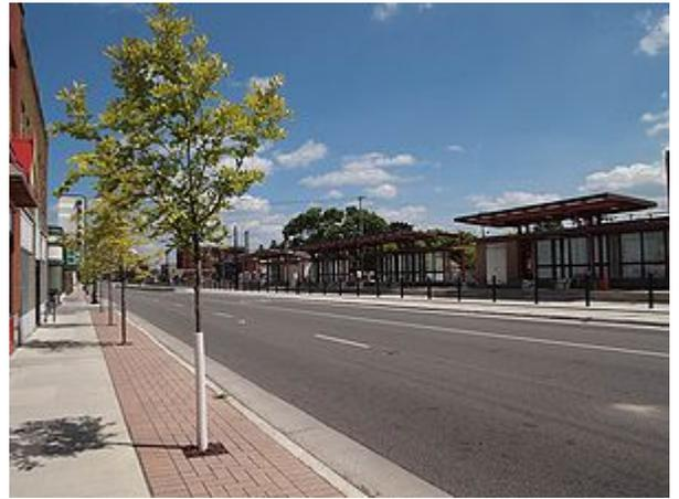
Photo of the completed tree system for the Central Corridor Light Rail Transit project, St. Paul, Minnesota. This system combines permeable pavement with a tree trench system. Image courtesy of the Capitol Region Watershed District (<http://www.capitolregionwd.org/>).
