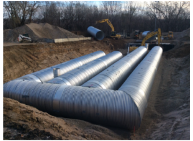
TrueNorthSteel infiltration system in native sandy soils
