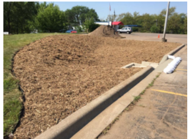
Infiltration basin before planting
