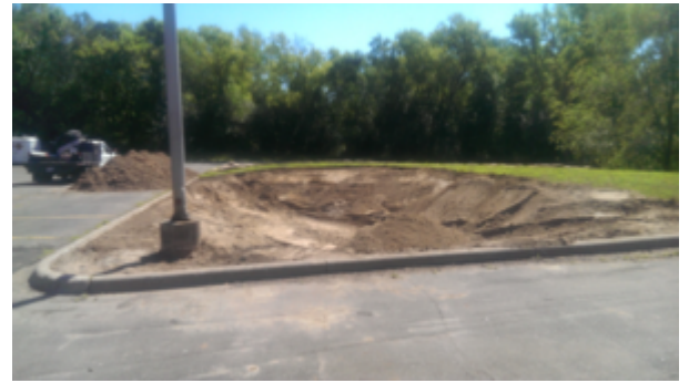
Infiltration basin with rough grading complete
