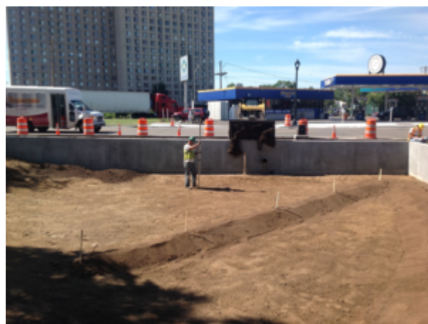
Infiltration soil being carefully placed to avoid compaction
