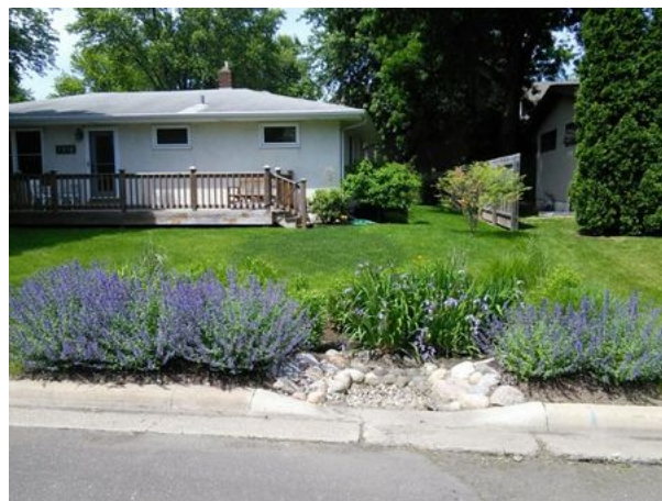
Bioinfiltration (rain garden) in a residential development. Photo courtesy of Katherine Sullivan.
