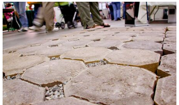
Permeable pavers let rain flow straight into the underlying soil
