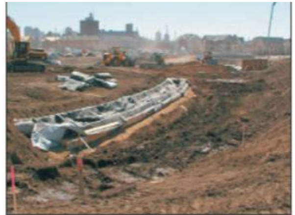
Photo illustrating the installation of a forebay.
