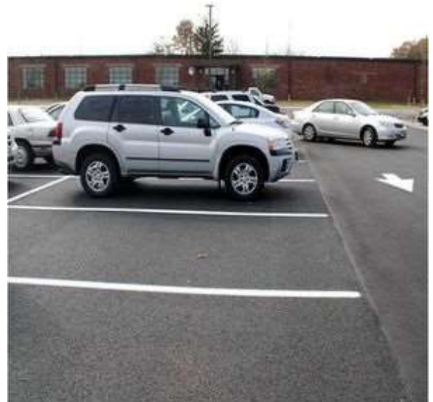
Photo illustrating porous asphalt. Porous asphalt is standard hot-mix asphalt that allows water to drain through it.
