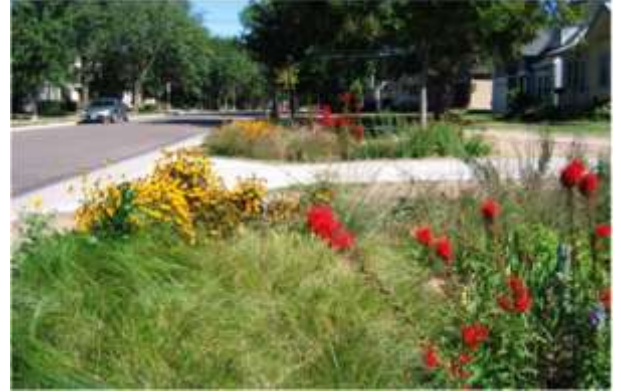
Bioretention practices can be incorporated into street landscapes. Image Courtesy of Emmons & Olivier Resources, Inc.
