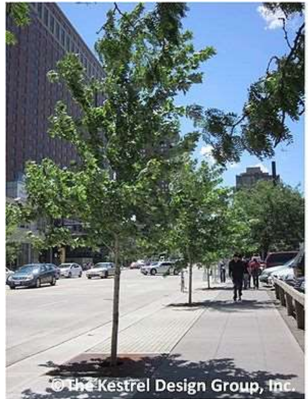
Completed tree system, Marquette and 2nd Avenue Busways project, Minneapolis, MN. Image Courtesy of The Kestrel Design Group.
