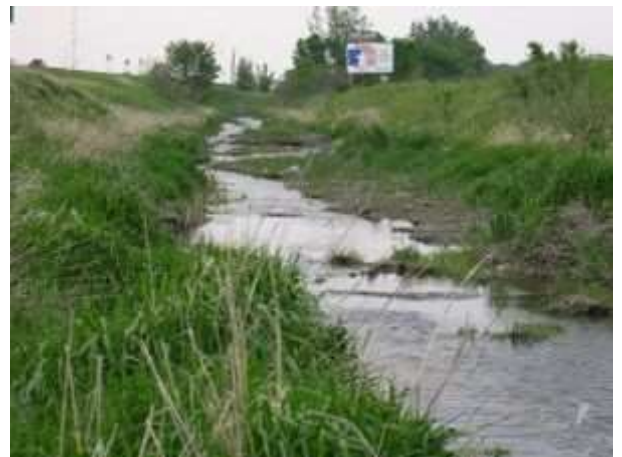
Photo of a wet swale. Courtesy of Limnotech.
