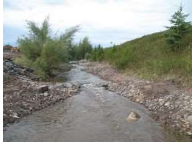
Stormwater step pool. Courtesy of Limnotech.
