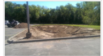
Infiltration basin with rough grading complete
