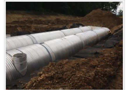
Installation of underground infiltration pipes.
