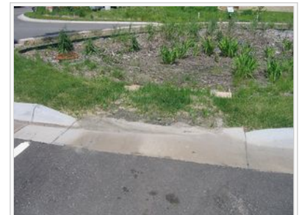
Maintenance of vegetated infiltration practices is critical during the establishment period. Although some plants look healthy in this photo, maintenance is needed to remove sediment from the filter strip and inflow area, remove weeds from the basin, re-
