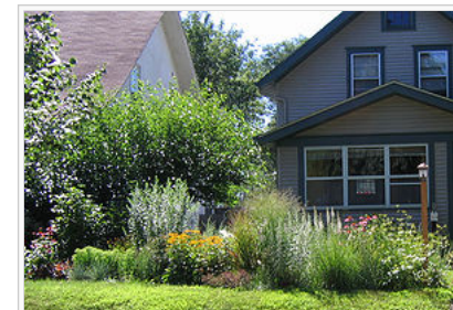
This bioretention basin utilizes several native species.
