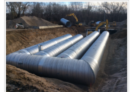
TrueNorthSteel infiltration system in native sandy soils
