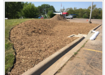
Infiltration basin before planting
