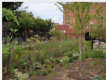
Bioinfiltration basin (Source: CDM Smith)
