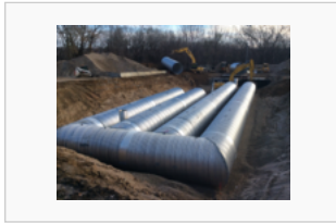
TrueNorthSteel infiltration system
