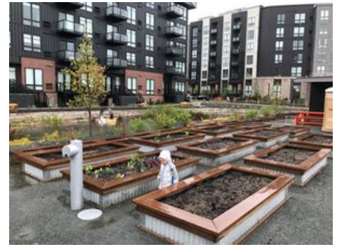
The Towerside District Stormwater System created a publicly accessible pocket park (rear) which integrates into and irrigates Minneapolis’s newest park and community garden (foreground).
