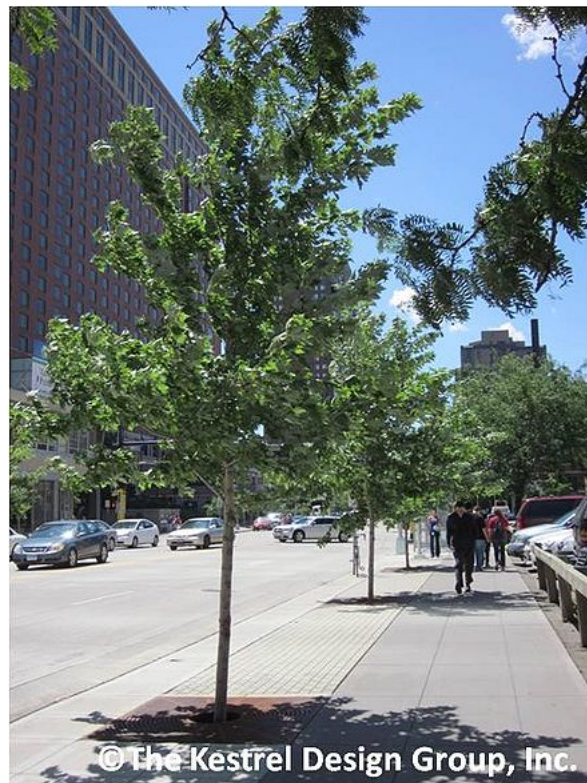
Completed tree system, Marquette and 2nd Avenue Busways project, Minneapolis, MN. Image Courtesy of The Kestrel Design Group.
