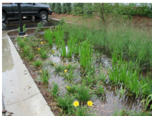
A properly functioning bioinfiltration practice should drain within 48 hours of a runoff event
