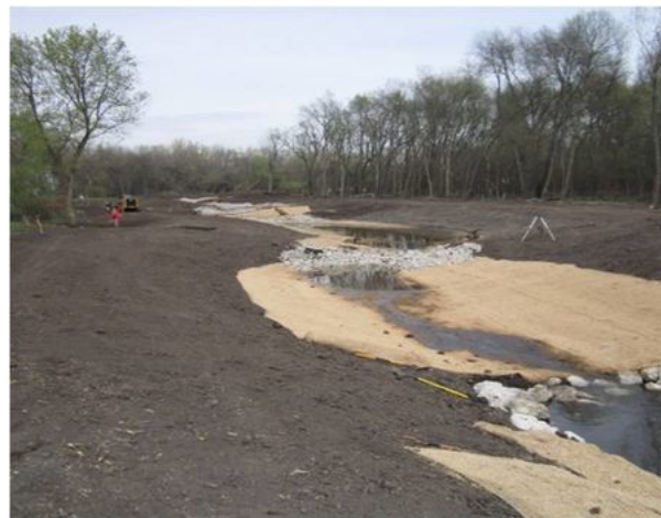
View of construction with erosion control.
