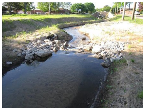
Views of the vane weir and riffle control structures installed.
