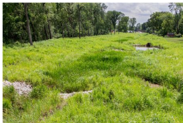
Views of the vane weir and riffle control structures installed.
