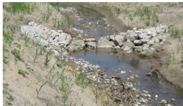
View of vane weir installed.
