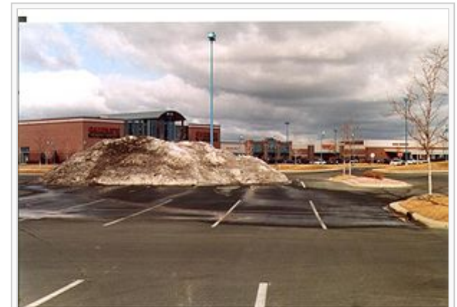
Snow plowed and piled in parking lot. Consideration should be given in locating these "snow dumps", since they will contribute a significant amount of stormwater runoff.
