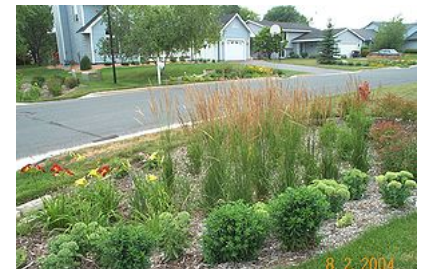
A well landscaped stormwater practice provides multiple benefits, such as pollinator habitat and aesthetic value, in addition to water quality and quantity benefits.
