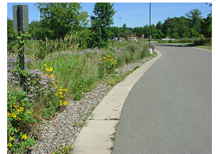
Photo of a Infiltration trench in Lino Lakes. This site illustrates how site aesthetics and landscaping are considered in the BMP design.
