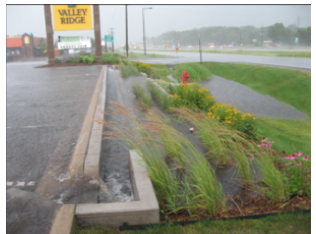
A properly functioning swale should drain within 48 hours of a runoff event
