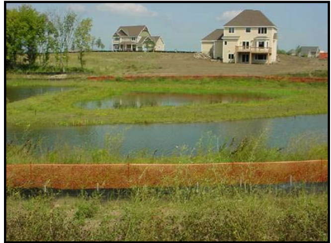
Site with temporary sediment control
