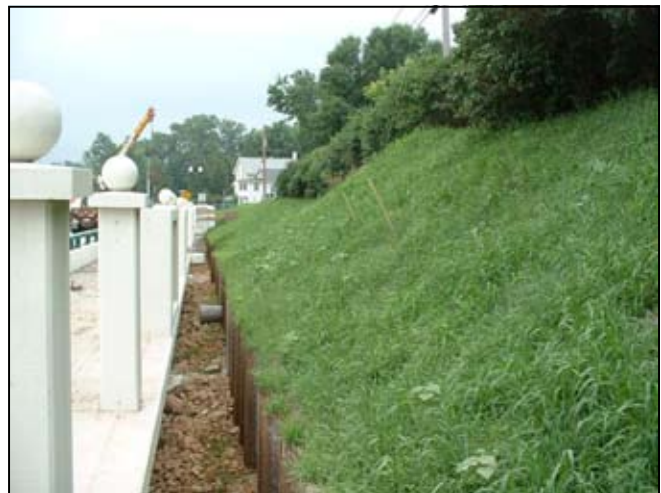
County Road 41 roadside in Carver County after application of compost blanket.
