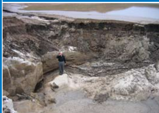
Figure 13.3 Calvin Alexander in Collapsed Karst Hole (Source: Kristin Daniels, 2005)
