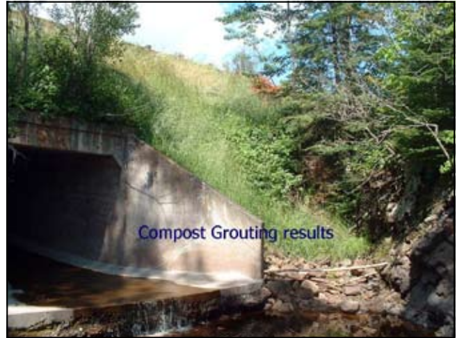
Highway 61 roadside after application of compost grouting.
