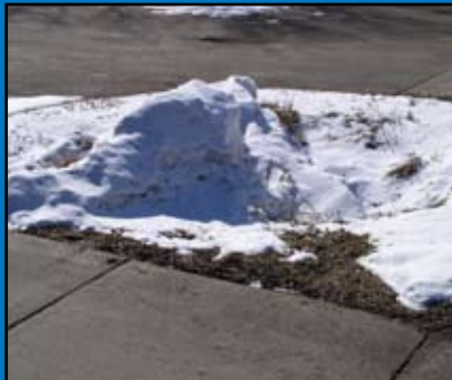
Figure 9.12b Snow Plowed Off Parking Lot Over Curb and Onto Grassy Depression
