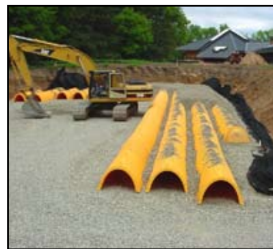
Bradshaw Celebration of Life Center - underground storage & infiltration Stillwater, MN
