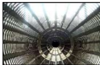
Gross Solids Removal Devices are BMPs that extend inlet pipes, dewater the inflow and leave the debris behind.
