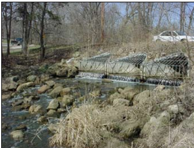
Highway drainage designers are ultimately left with the task of capturing runoff that does not infiltrate and then routing it via stormsewer to an outlet
