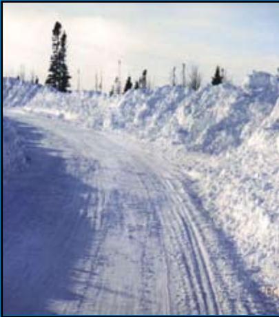
Figure 9.6a Snow Plowed Off the Road and Left Piled on the Roadside
