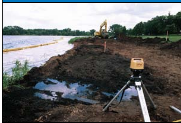
Figure 14.32 West Shore Excavation
