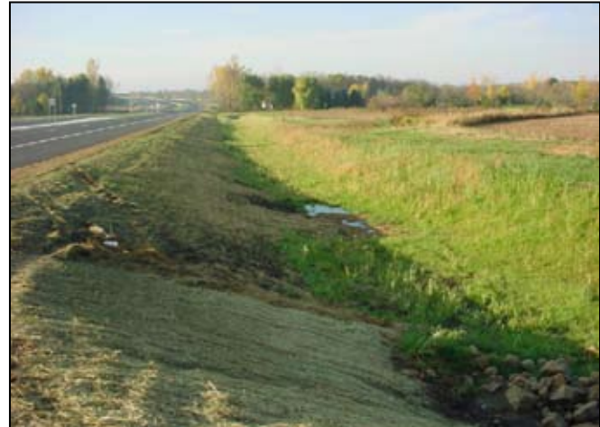
A well drained swale can be a very effective BMP for both reducing volume through infiltration and for improving water quality through filtration, settling and vegetative uptake.
