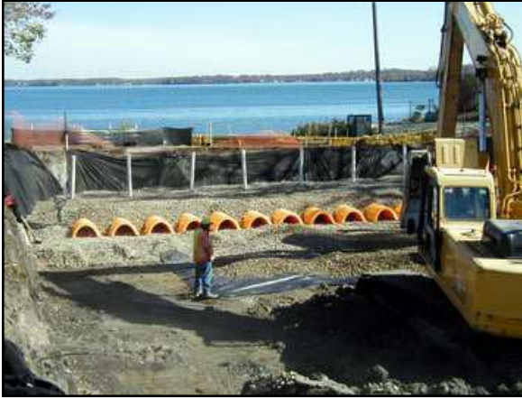
Figure 14.24 Filtration System Installation
