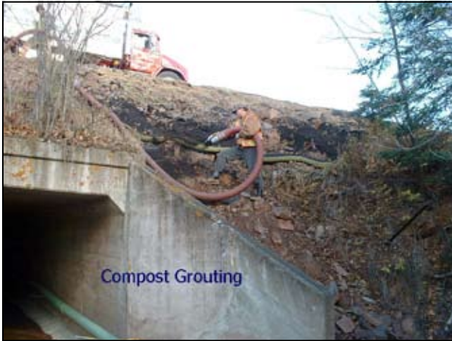
Compost grouting on Highway 61.
