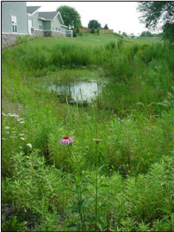
Math & Science Academy - infiltration trench Woodbury, MN
