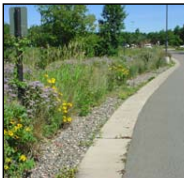
Lino Lakes City Hall - Infiltration trench Lino Lakes, MN
