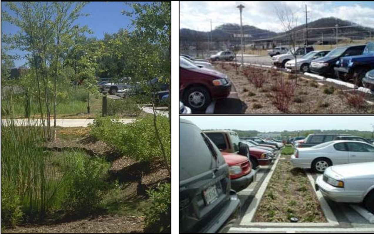
Figure 4.5 Examples of the Use of Landscaped Islands for Stormwater Treatment in a Suburban Parking Lot (left), the Parking Lot of a Government Office Building (right top), and a Highly Urban Parking Lot (right bottom)
