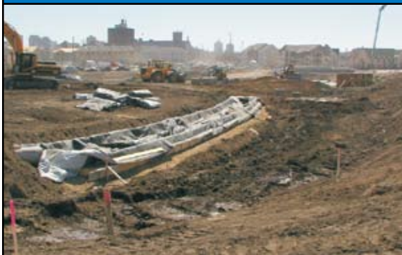
Figure 14.7 Installation of Trench Forebay
