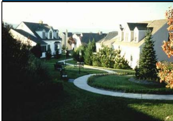
Figure 4.7 Sidewalk that Drains to Adjacent Vegetation and Provides Common Walkways Linking Pedestrian Areas
