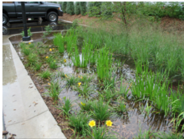
A properly functioning bioretention practice should drain within 48 hours of a runoff event
