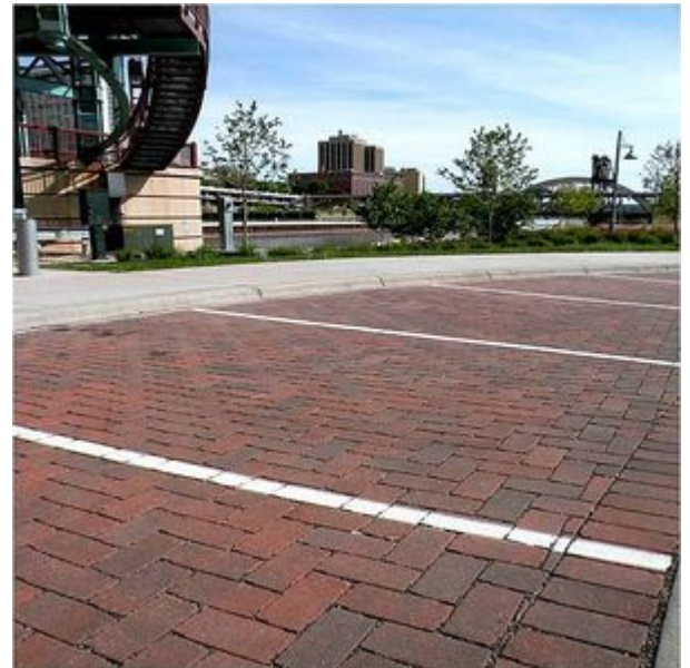
Photo illustrating permeable interlocking concrete pavement.
