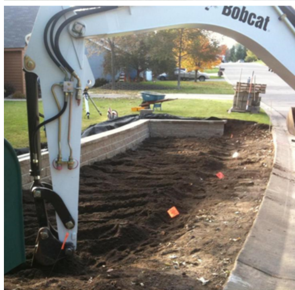
Example of subsoiling and incorporation of compost and sand. Note the equipment is kept out of the practice.
