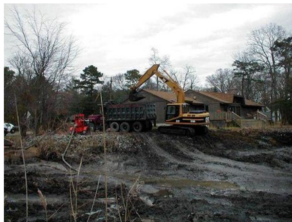
Example of a site where vehicle traffic occurred within the infiltration practice, resulting in soil compaction and ponding of water.
