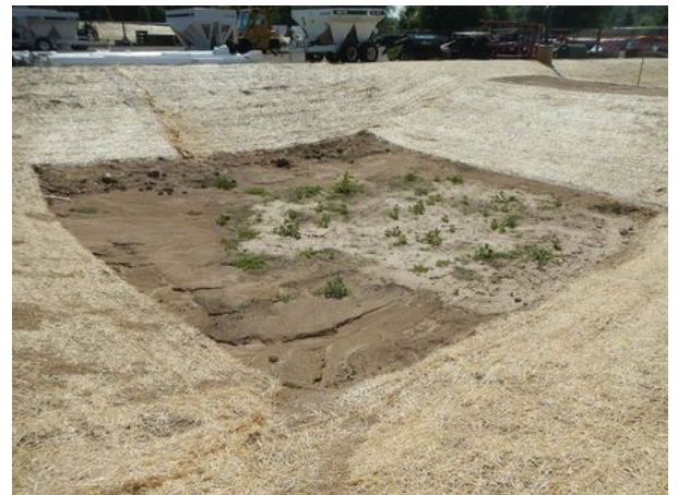
Sparse vegetation and erosion within an infiltration basin may be an indicator of compacted soils.
