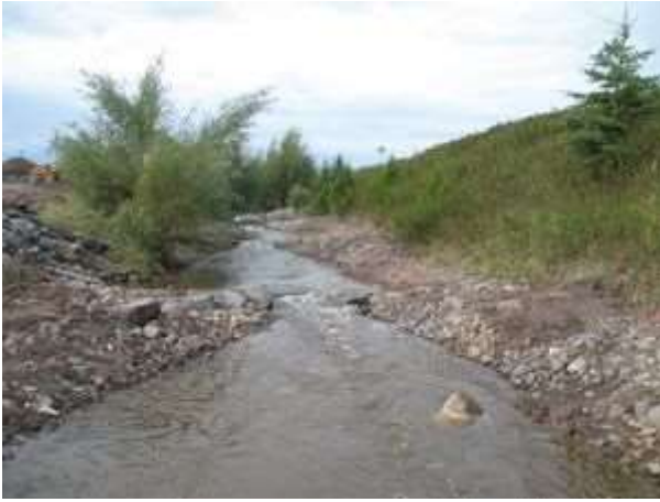
Stormwater step pool. Courtesy of Limnotech.
