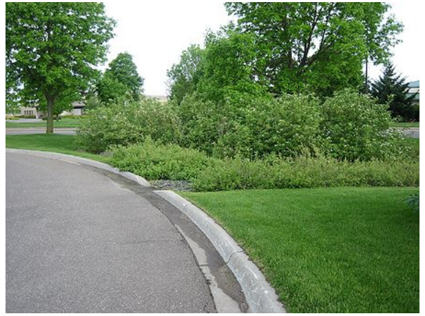
A bioretention facility (rain garden) in a residential area. Note the curb cut that allows water to enter the facility.
