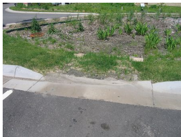
Image of a vegetated filter strip
