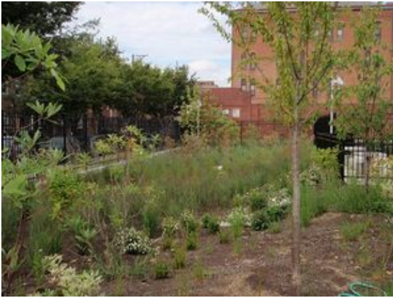
Bioinfiltration basin (Source: CDM Smith)
