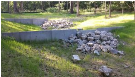
Dry swale with impermeable concrete check dams. Photo courtesy Limnotech.
