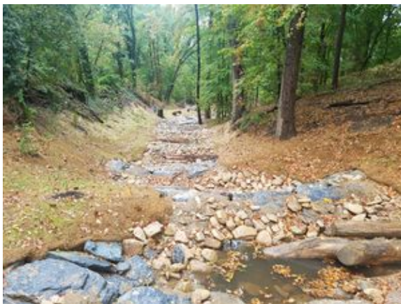
Step pool with impermeable check dam. Courtesy of Limnotech.
