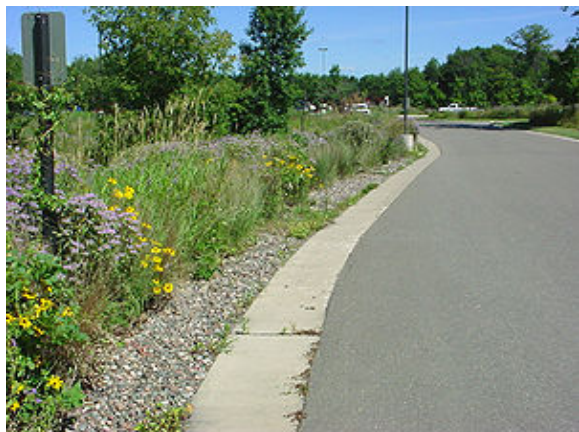
Photo of a Infiltration trench in Lino Lakes
