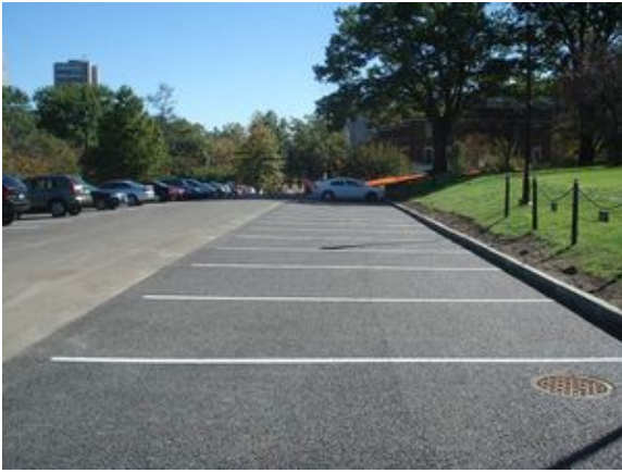
Permeable pavement (Source: CDM Smith)
