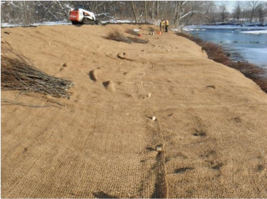
Woven 100% natural fiber erosion-control materials. Photo by Nick Proulx courtesy of MN DNR.
