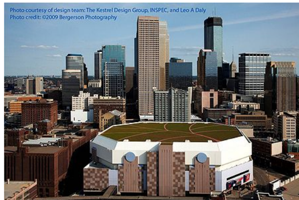
View of the Target Center Arena green roof, located in downtown Minneapolis, Minnesota. Image by Bergerson Photography, Courtesy of The Kestrel Design Group, Inc., INSPEC, and Leo A Daly.
