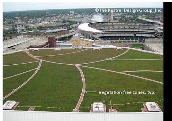
Vegetation free zones at Target Center Green Roof, Minneapolis, MN. Image courtesy of The Kestrel Design Group, Inc.
