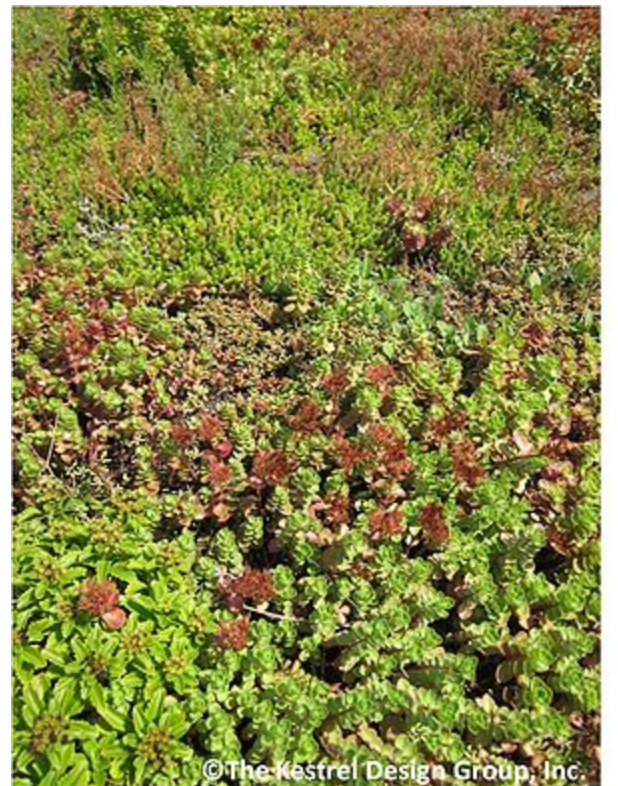
Photo of sedums on the Target Center Arena green roof in Minneapolis, MN. Sedums are relatively tolerant of dry conditions. Image Courtesy of The Kestrel Design Group, Inc.
