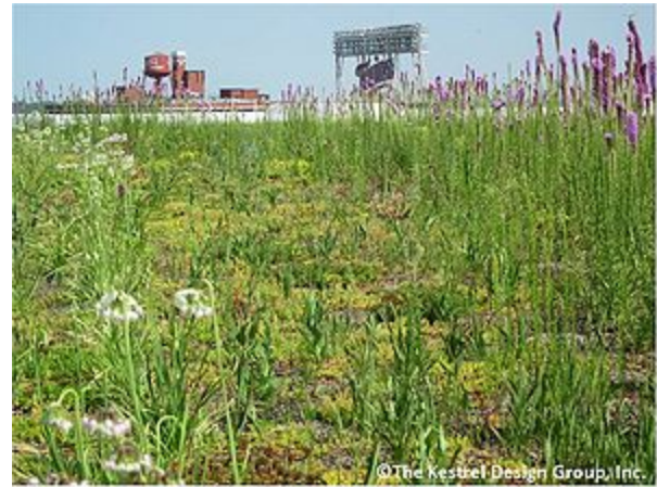
Native Plants on Target Center Arena Green Roof, Minneapolis, MN. Image Courtesy of The Kestrel Design Group, Inc.
