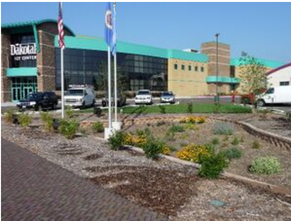
Dakotah! Ice Center permeable pavers and rain garden
