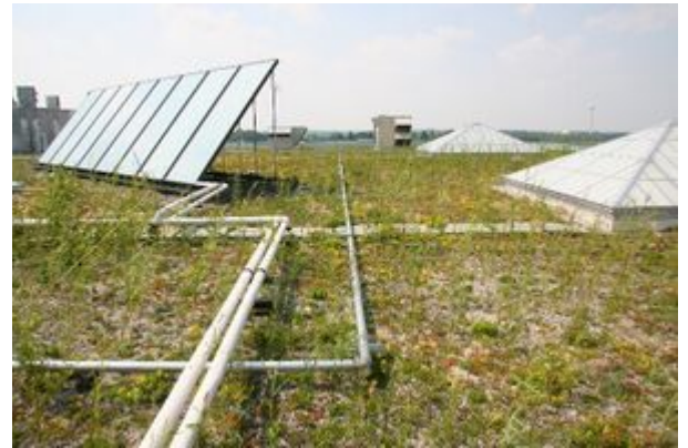
Finished green roof with solar panels
