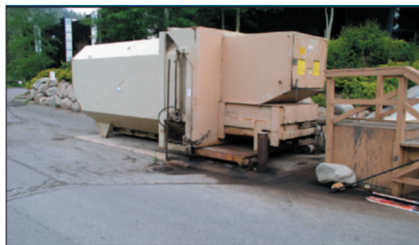
Dumpster leaking directly into a storm sewer.
