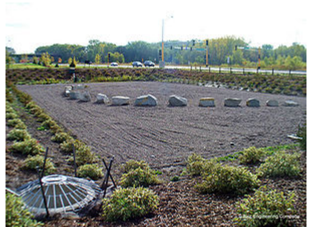
Iron enhanced sand filter basin, Maplewood, MN. Photo courtesy of Barr Engineering.
