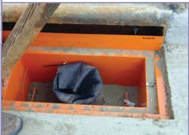
A street view and the inside of one type of inlet protection device.
