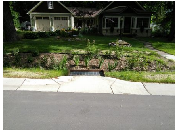
Pretreatment screen for a residential raingarden. Photo courtesy of Katherine Sullivan.
