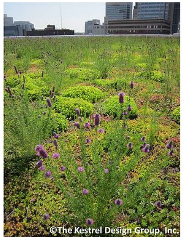
Photo showing the sedum mat with additional plants. Image Courtesy of The Kestrel Design Group, Inc.
