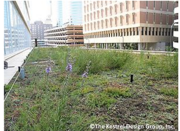
Minneapolis Central Library 2nd floor south facing green roof, Minneapolis, MN. Image Courtesy of The Kestrel Design Group, Inc.
