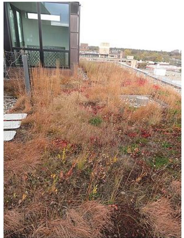
Edgewater green roof in late summer. Image Courtesy of The Kestrel Design Group, Inc.
