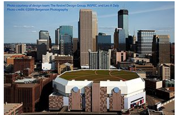
View of the Target Center Arena green roof, located in downtown Minneapolis, Minnesota. Image by Bergerson Photography, Courtesy of The Kestrel Design Group, Inc., INSPEC, and Leo A Daly.
