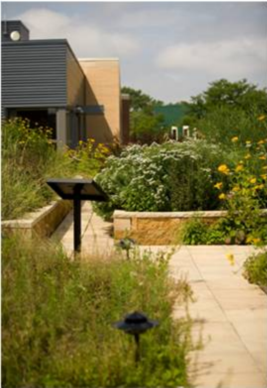
St Paul Firestation green roof, illustrating vegetation-free zones and walking paths with informational kiosks. Image Courtesy of Angie Durhman, AD Greenroofs
