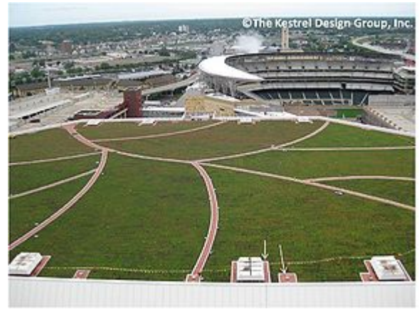
Aerial view of the Target Center Arena green roof, showing vegetation-free zones and some of the patterns incorporated into the roof for aesthetic purposes. Image Courtesy of The Kestrel Design Group, Inc.
