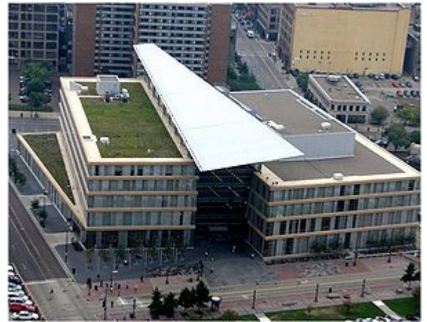
Minneapolis Central Library aerial view of south facing 2nd floor roof and 5th floor roof green roof, Minneapolis, MN.
