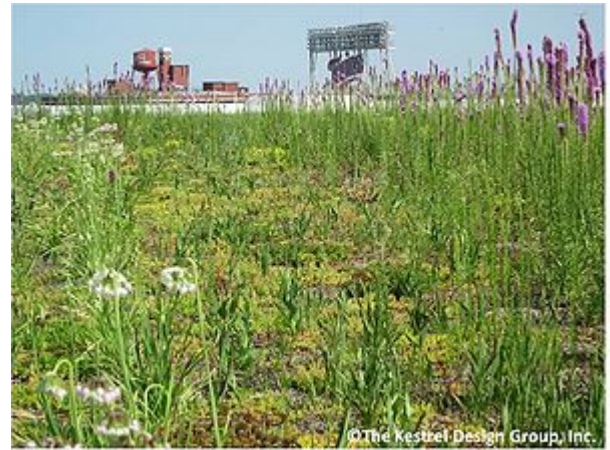
Vegetation on the Target Center Arena green roof. vegetation consisted of a pre-grown Sedum mat supplemented with 22 species of plugs and 16 species of seed native to Minnesota's bedrock bluff prairies. Image Courtesy of The Kestrel Design Group, Inc.
