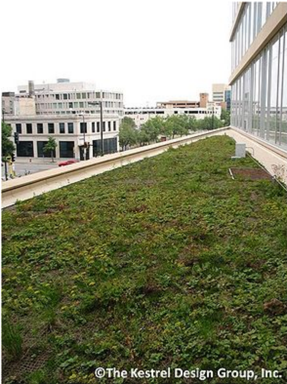
Minneapolis Central Library 2nd floor northwest facing green roof, Minneapolis, MN. Image Courtesy of The Kestrel Design Group, Inc.
