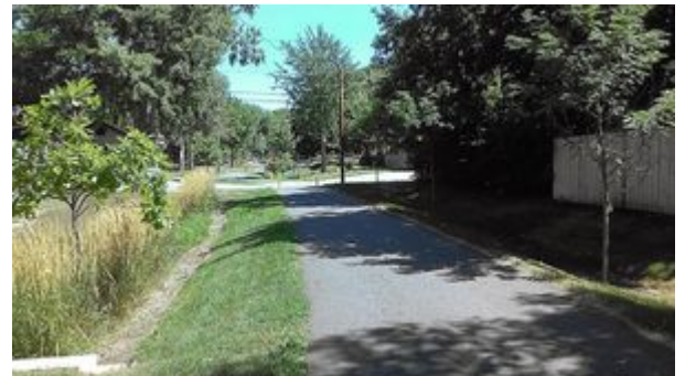
The vegetated filter strip in this photo is pretreatment for a bioswale. Photo courtesy of Alisha Goldstein, U.S. EPA.
