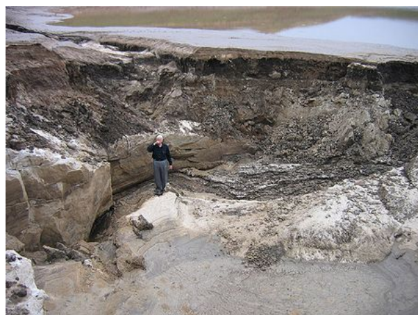
Woodbury sinkhole collapse looking toward the south.
