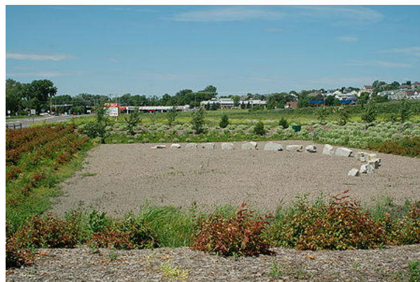
Iron enhanced sand filter basin, Maplewood, MN. Photo courtesy of Ramsey-Washington Watershed District.
