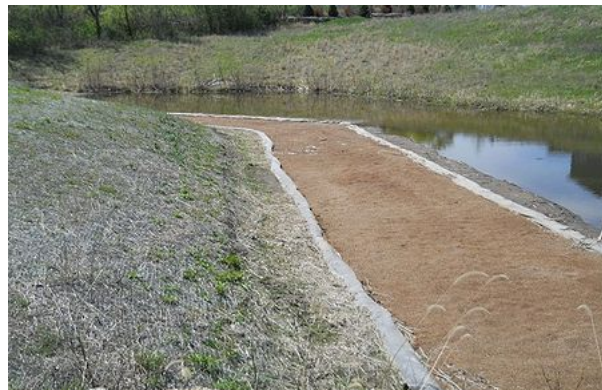
Iron enhanced sand bench, Prior Lake, MN. Photo courtesy of Ross Bintner.
