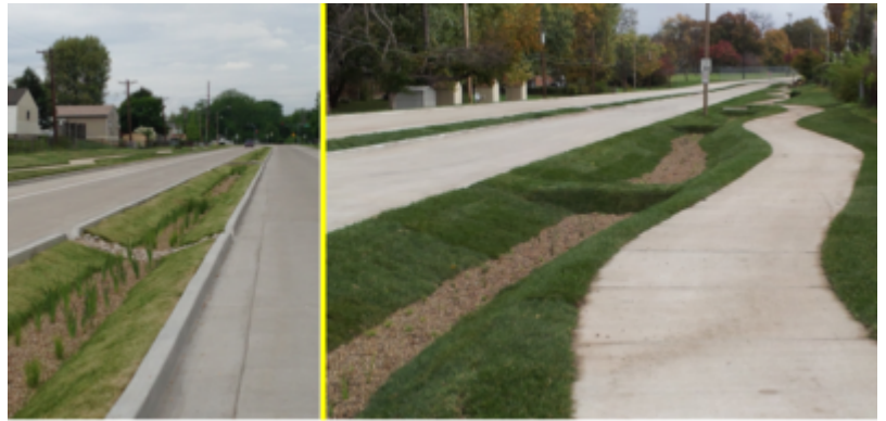
View of constructed median and road-adjacent dry swales.
