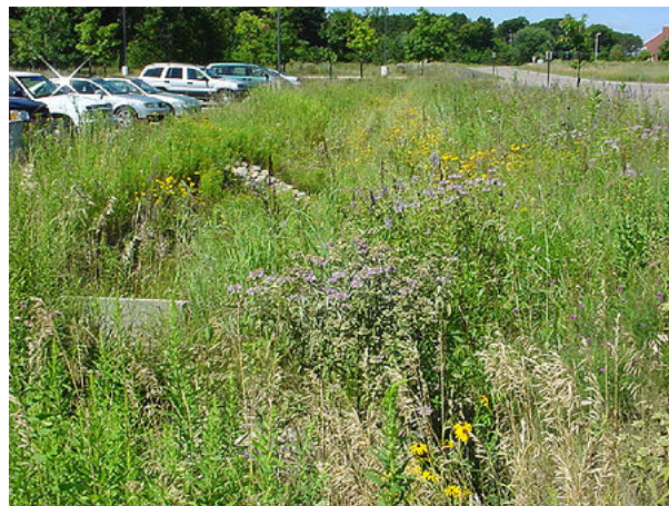
Image of a swale at Lino Lakes city hall
