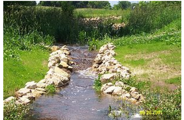
Photo showing a reinforced vegetated conveyance
