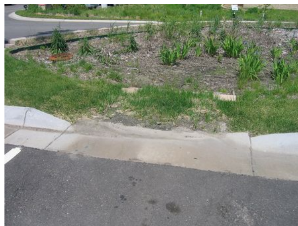
Image of a vegetated filter strip
