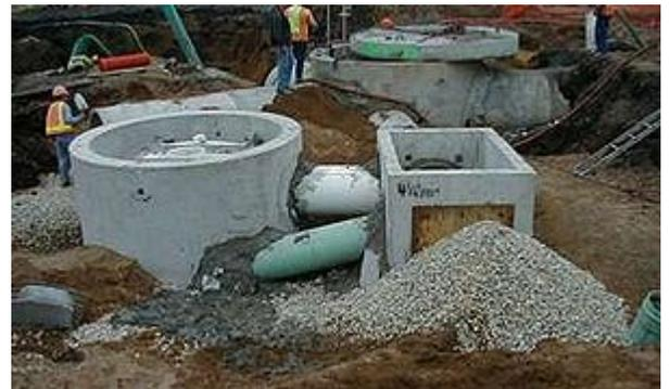
Photo showing installation of grit chamber
