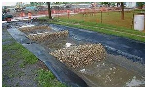
Photo illustrating a temporary sedimentation basin
