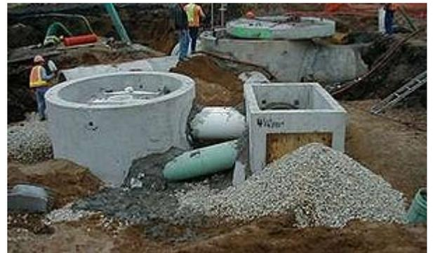
Photo showing installation of grit chamber
