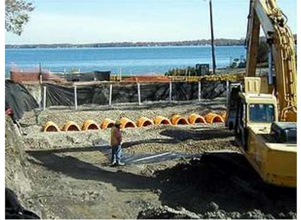
Photo illustrating installation of a filtration system
