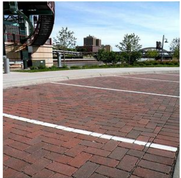
Photo illustrating permeable interlocking concrete pavement. Permeable interlocking pavers consist of concrete or stone units with open, permeable spaces between the units.
