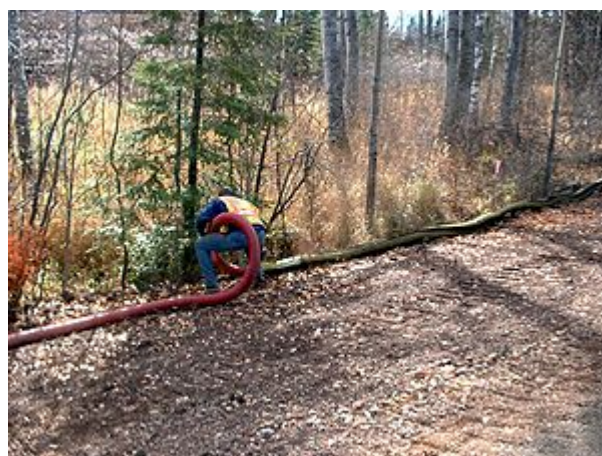
Photo illustrating perimeter control using compost filter logs.
