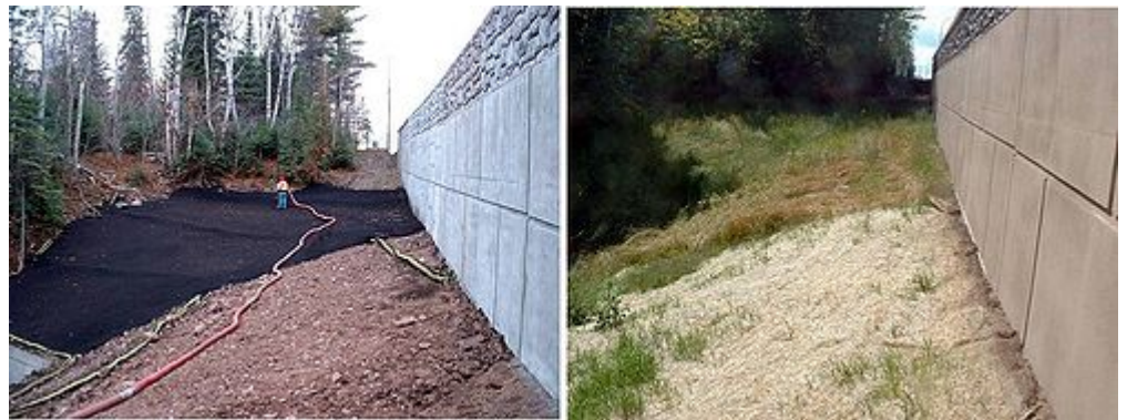
Photo showing stabilization and revegetation using compost vegetated mat (a) installation and after stabilization (b). Note that areas utilizing compost vegetated more quickly and completely than areas using the vegetative mat.
