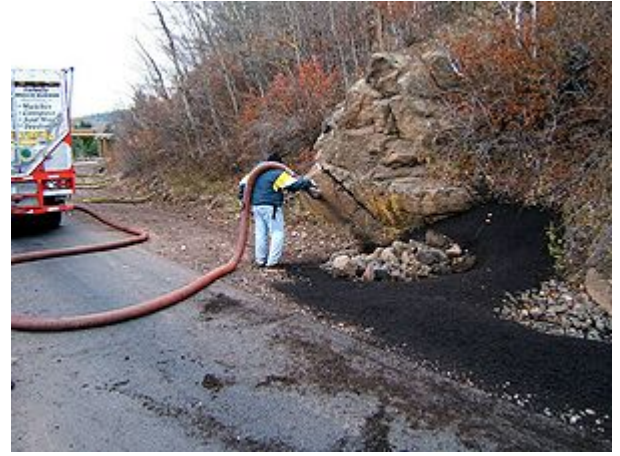
Photo showing addition of a soil amendment for rapid vegetation and stabilization.
