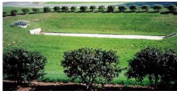
Photo of a dry pond
