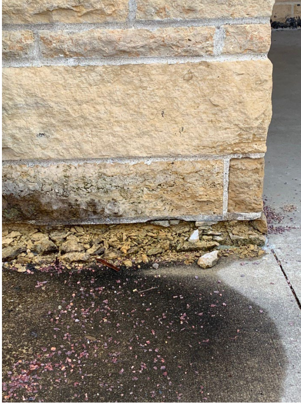
Infrastructure damage due to salt. Image courtesy of Nick Queensland.
