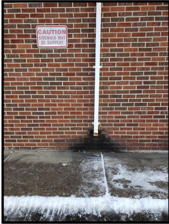
Downspout directing roof melt to sidewalk creating unsafe conditions and the excessive use of salt. Images courtesy of Bolton & Menk.
