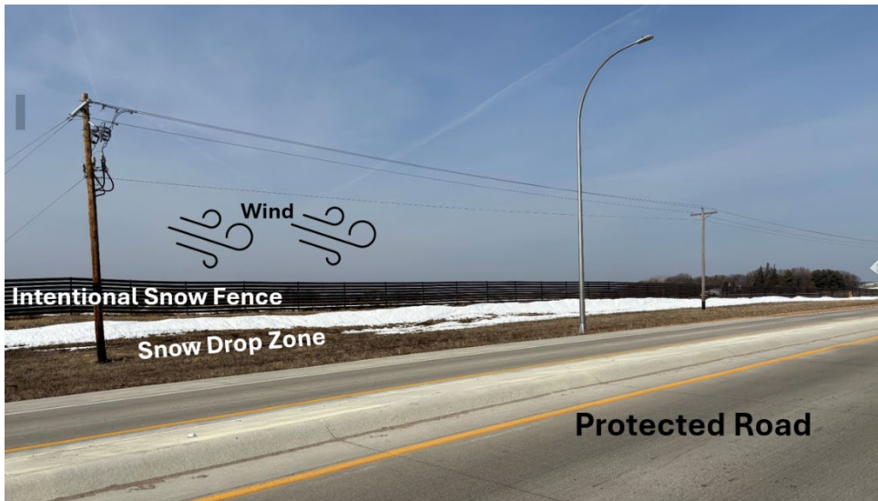
Success! Effective sequence from left to right: wind, snow fence, snow drop zone, protected road. Image courtesy of Bolton & Menk.
