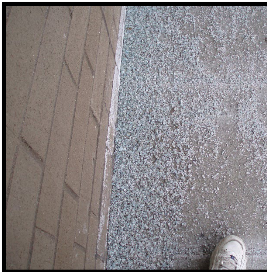
The image on the left reflects the problem caused by dripping snowmelt. The image on the right shows excessive salt use near the building where vertical drainage is a problem. Image courtesy of Bolton & Menk (Left) and Jenny Winkleman (Right).
