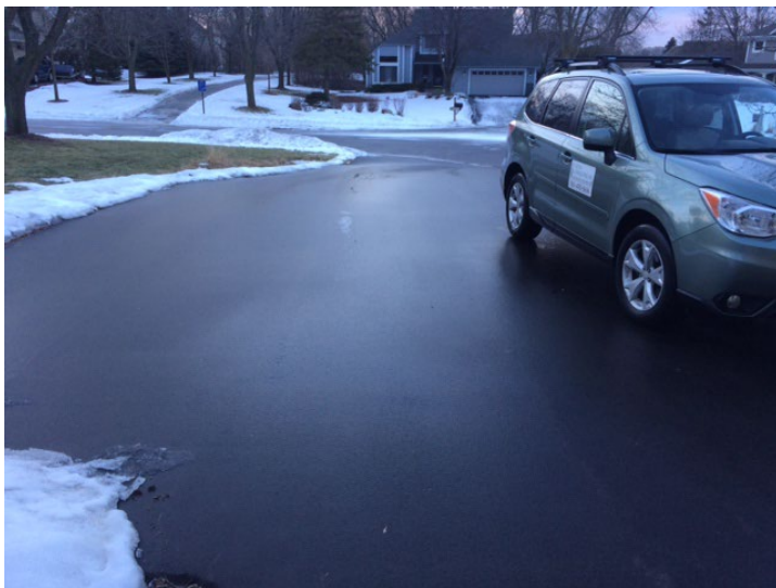
Wet pavement from a winter rain event: This cannot be controlled in design to prevent a sheet of ice unless more drastic measures are employed such as heated pavement or covered surfaces. Image courtesy of Bolton & Menk.
