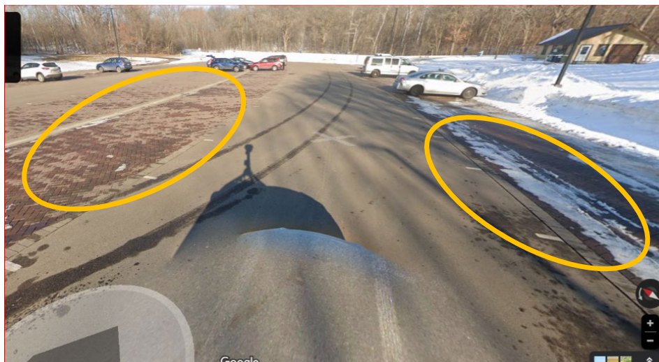
Permeable pavers placed in the sun provide winter benefit in addition to summer benefit. Permeable pavers in the shade show reduced winter benefit. Image courtesy of Google Earth.
