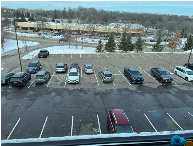
Superelevated surfaces have a high risk of meltwater sprawl. Image courtesy of Bolton & Menk.
