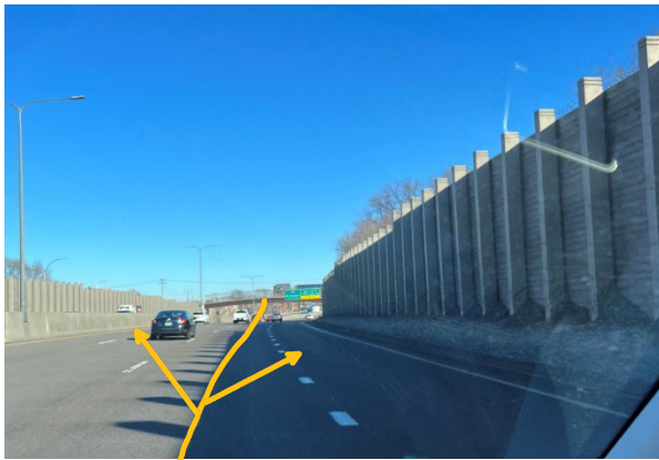
The left side has faster pavement recovery. The right side has slower pavement recovery. Image courtesy of Bolton & Menk.
