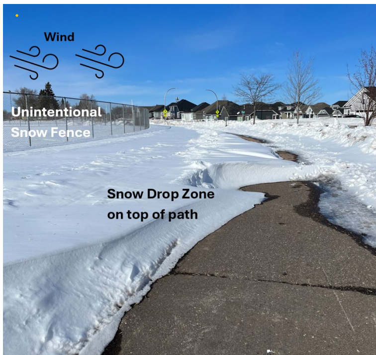
Failure! Ineffective sequence from left to right: wind, unintentional snow fence, drop zone on top of path. Image courtesy of Bolton & Menk.
