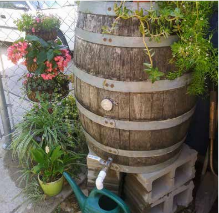
This home rain barrel in Mankato collects water from half of a garage roof and only takes a quarter inch of rain to fill. The barrel was raised off the ground to fit a watering can underneath the spigot and dressed up with plants which are watered with rain barrel water. Photo courtesy of Joanne Boettcher, MPCA.
