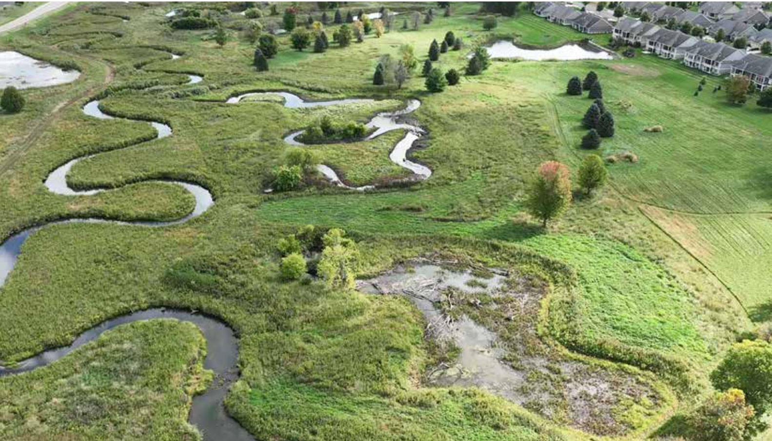
Years ago, Cascade Creek was forced into a straight channel through a former golf course in Rochester. The straight channel was stuck in its deep banks with fast flowing water that added to downstream flooding problems. The City of Rochester, Minnesota Department of Natural Resources, Olmsted County Soil and Water Conservation District (SWCD), and Minnesota Board of Water & Soil Resources collaborated to fund constructed wetlands, wetland restoration, and stream and prairie restoration on this 29-acre site.
