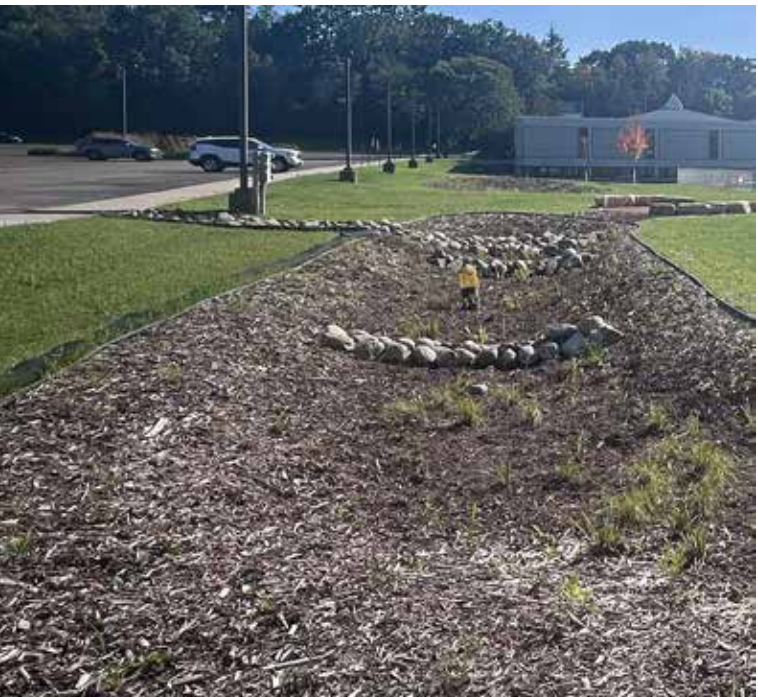
The recently completed rain garden at the Presbyterian Church of the Way in Shoreview was planted with plugs. Water enters from the parking lot through a rock channel. Rock strips are used in strategic places in the rain garden to help slow and filter runoff before entering the outlet structure, which is elevated and covered with a yellow grate. Photo courtesy of Kendra Sommerfield, Rice Creek Watershed District.
