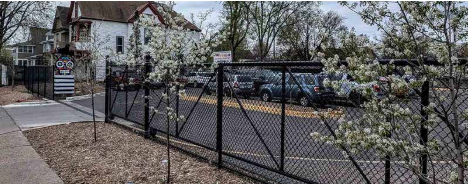
The old parking lot surface was removed at Mercado Central, leaving a rough construction site before the new project features were installed (top). About a year after the project was completed, the rain garden (background) is helping clean water, while the row
